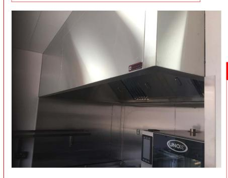
Vortex designed, manufactured and installed a bespoke extract canopy and extraction system at Bibby Financials new staff canteen in Banbury. The extraction included fire rated ductwork and discharge acoustic louvre.
