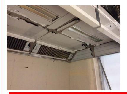
Vortex designed, manufactured and installed a bespoke extract and supply air canopy at Ole & Steen's new site in Oxford. The canopy had to be mounted over 2.5m high ovens and incorporate a safe access walkway for maintenance / cleaning of the associated ductwork/plant.
